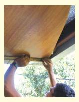
4.1 Once the Rustic is placed, fasten it to the frame skeleton by placing a fourth round board on top so that the board acts as a support and pressing at the same time; therefore, you can handle the Rustic and get the required position.
