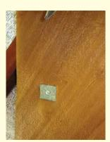
4.2 Use the head screws for the ceilings or build small 1" x 1 " tin squares to fasten the insulation to the wood of the frame skeleton across the structure. Remember that you will have flexibility with the placement of the Rustic.
