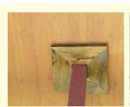
7.1 With 2" boards, make a square with cuts at 45 degrees and fasten them to the ceiling structure.
