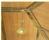
Install the lights using pipes or chutes; you can dye them using the same color of the wood to give a better appearance to the electrical installation.
